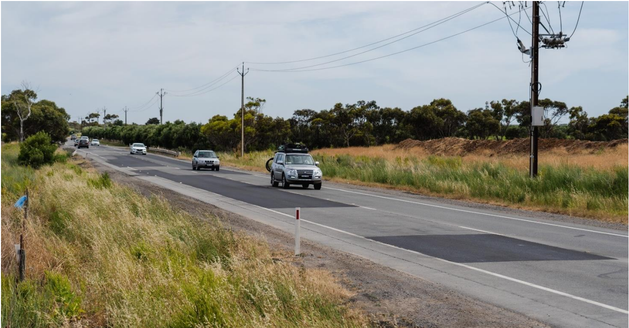
Figure 9: Most failures were repaired in late November, whilst the Risky Roads survey was still open
