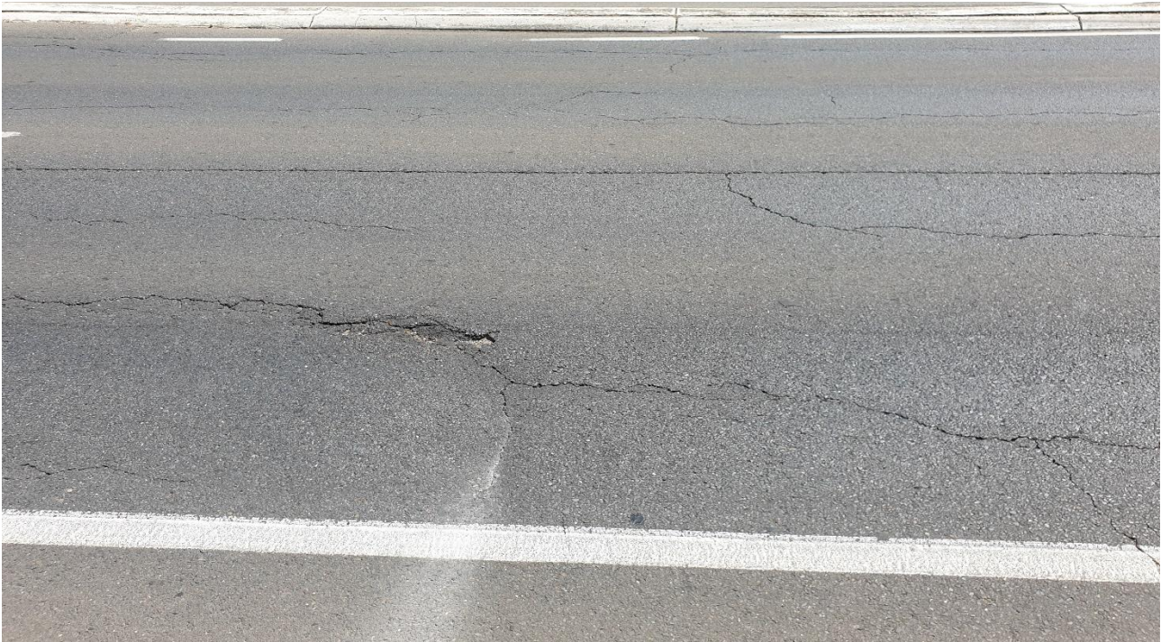
Figure 36: Cracks and a pothole forming on Grand Junction Road in Northgate
