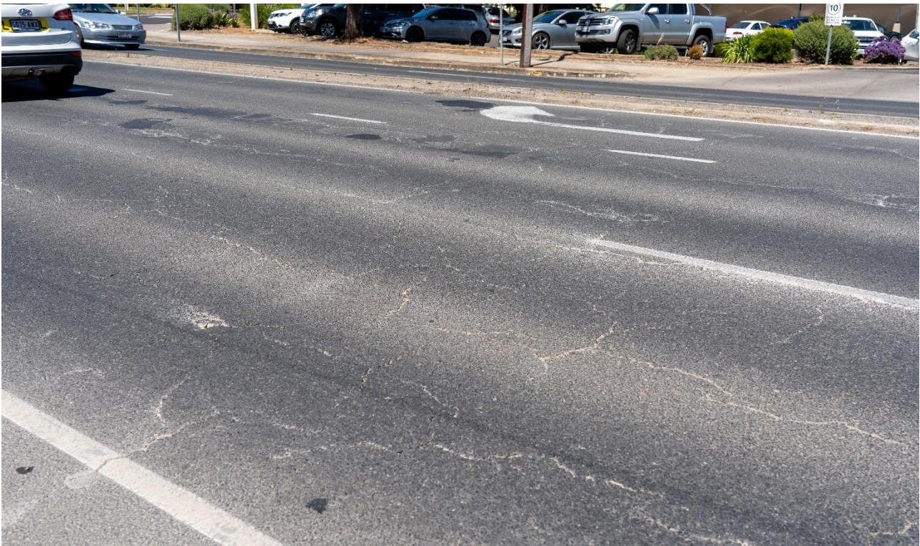
Figure 19: Cracking, ruts and potholes present on Glynburn Road near Firle Plaza
