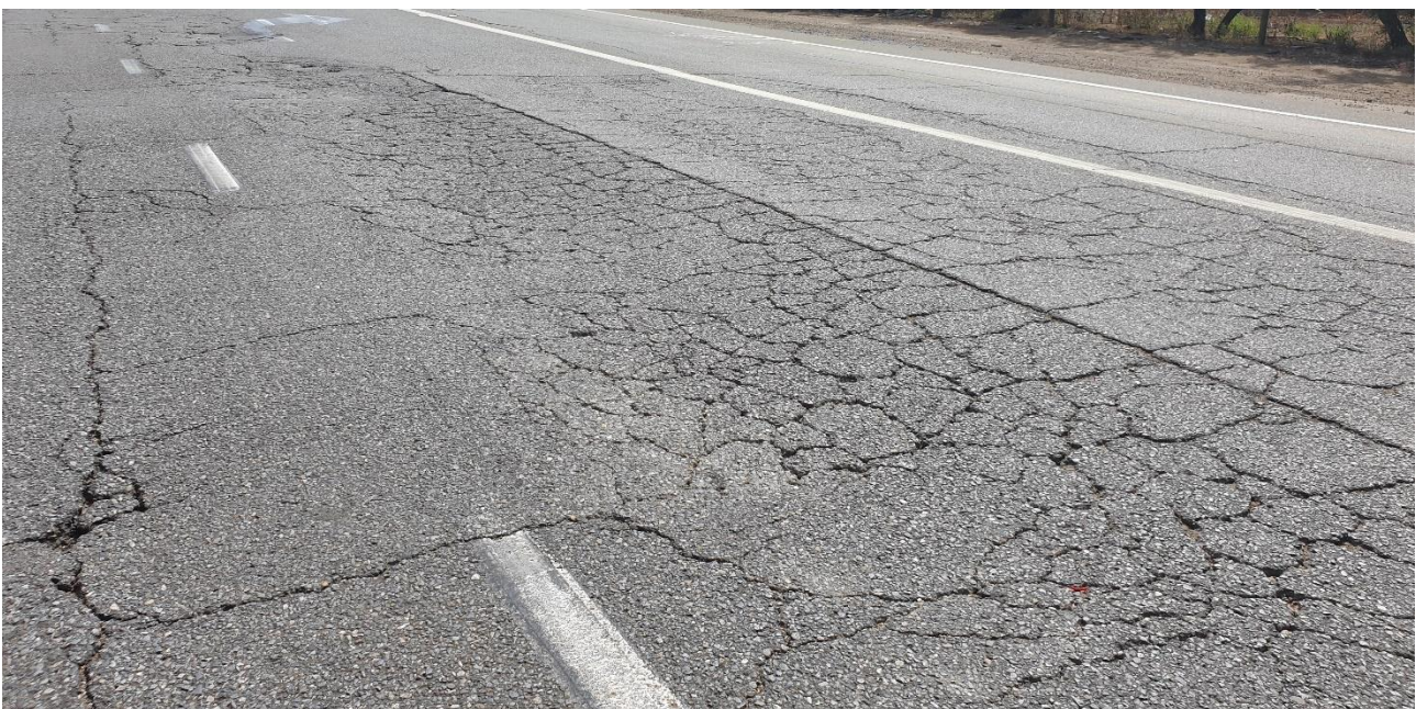
Figure 30: Cracks and rutting on Heaslip Road
