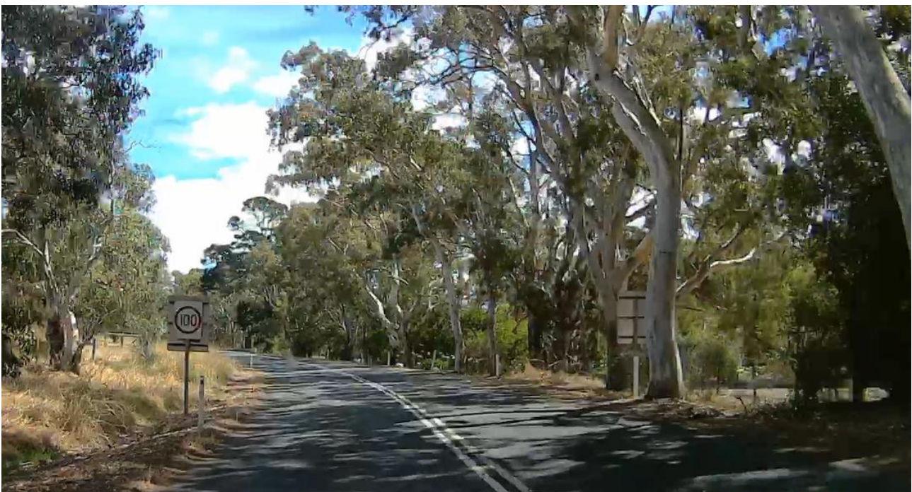
Figure 55: Inman Valley Road is narrow with a high speed limit and unforgiving roadsides.
