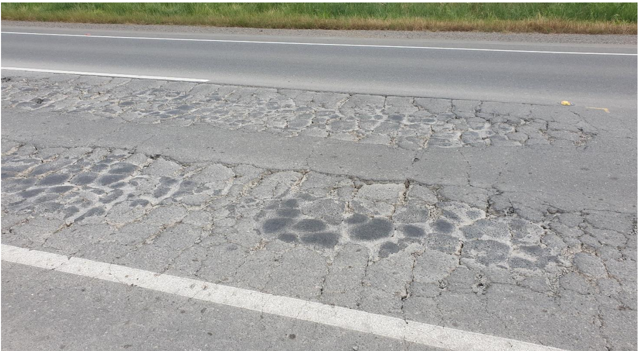
Figure 8: Major pavement failures on Main South Road between Aldinga and Sellicks Beach in November 2020
