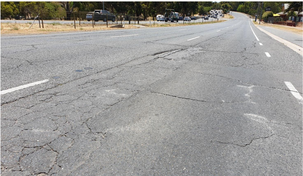
Figure 16: Deteriorating surface of Main North Road in Hillbank
