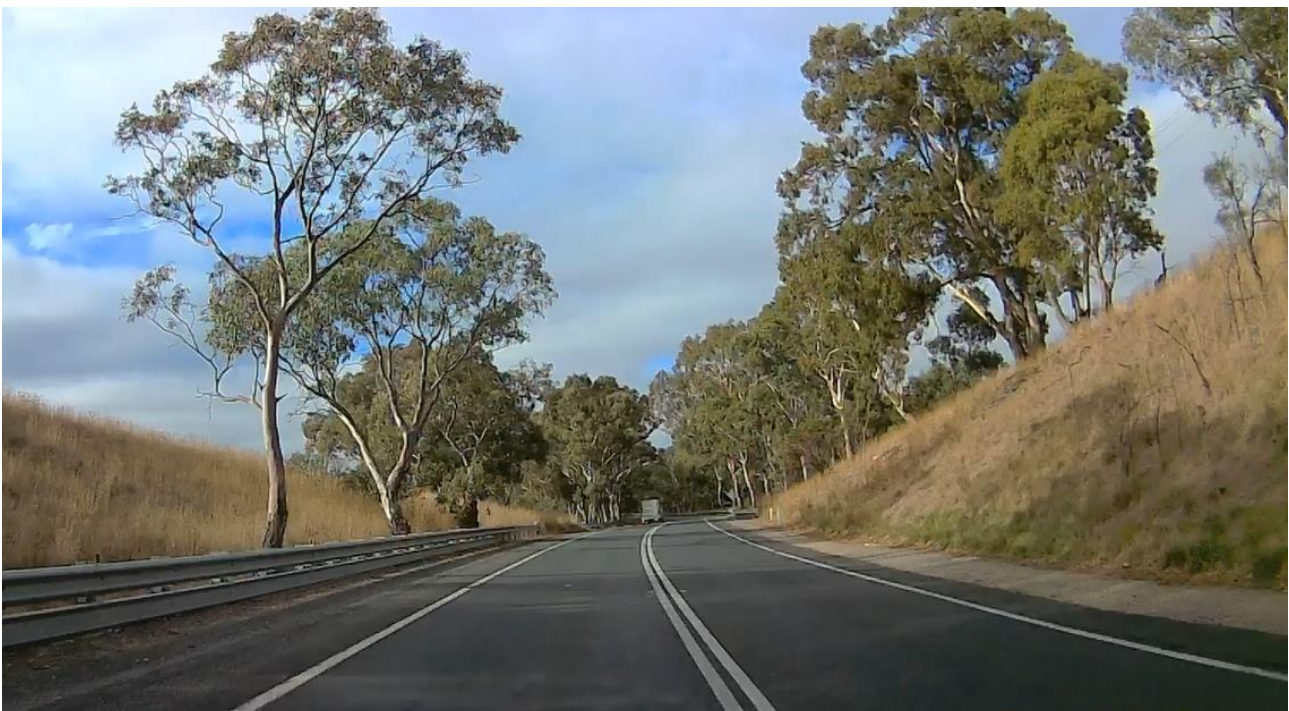
Figure 58: Overtaking opportunities are scarce on Long Valley Road due to curves and crests and high traffic volumes
