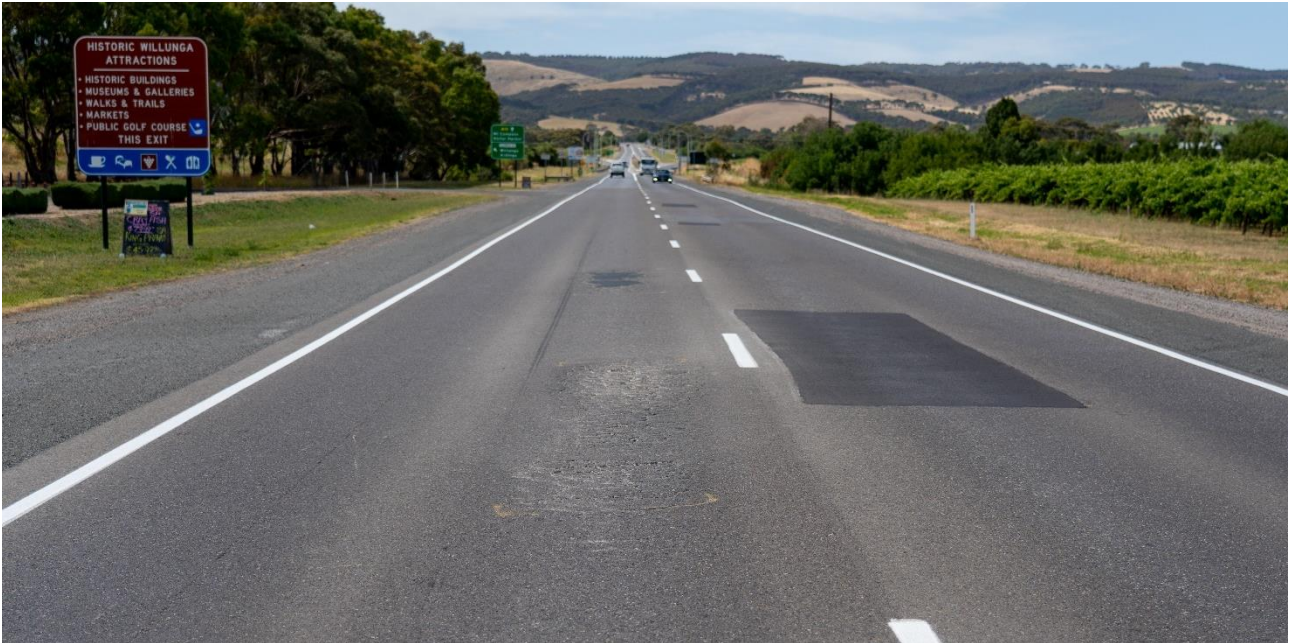
Figure 46: Sections of Victor Harbor Road between McLaren and Willunga are in poor condition
