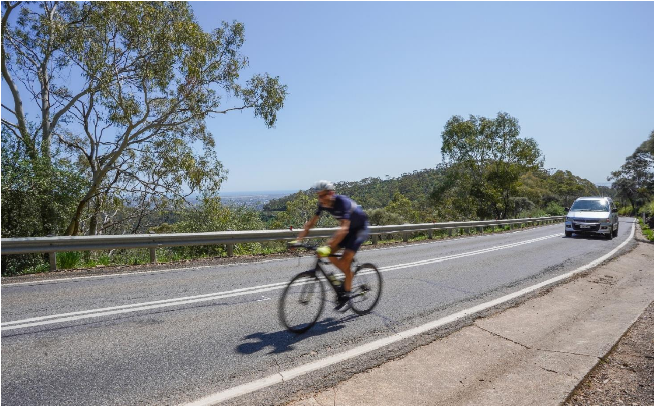
Figure 27: Greenhill Road is a narrow corridor, and popular with cyclists
