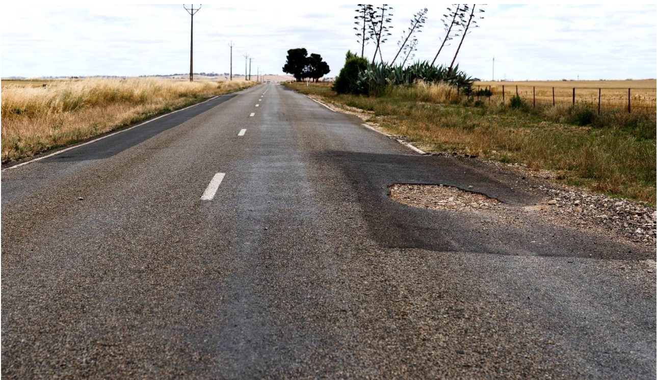
Figure 51: Previous minor repairs have not held up well along Owen Road
