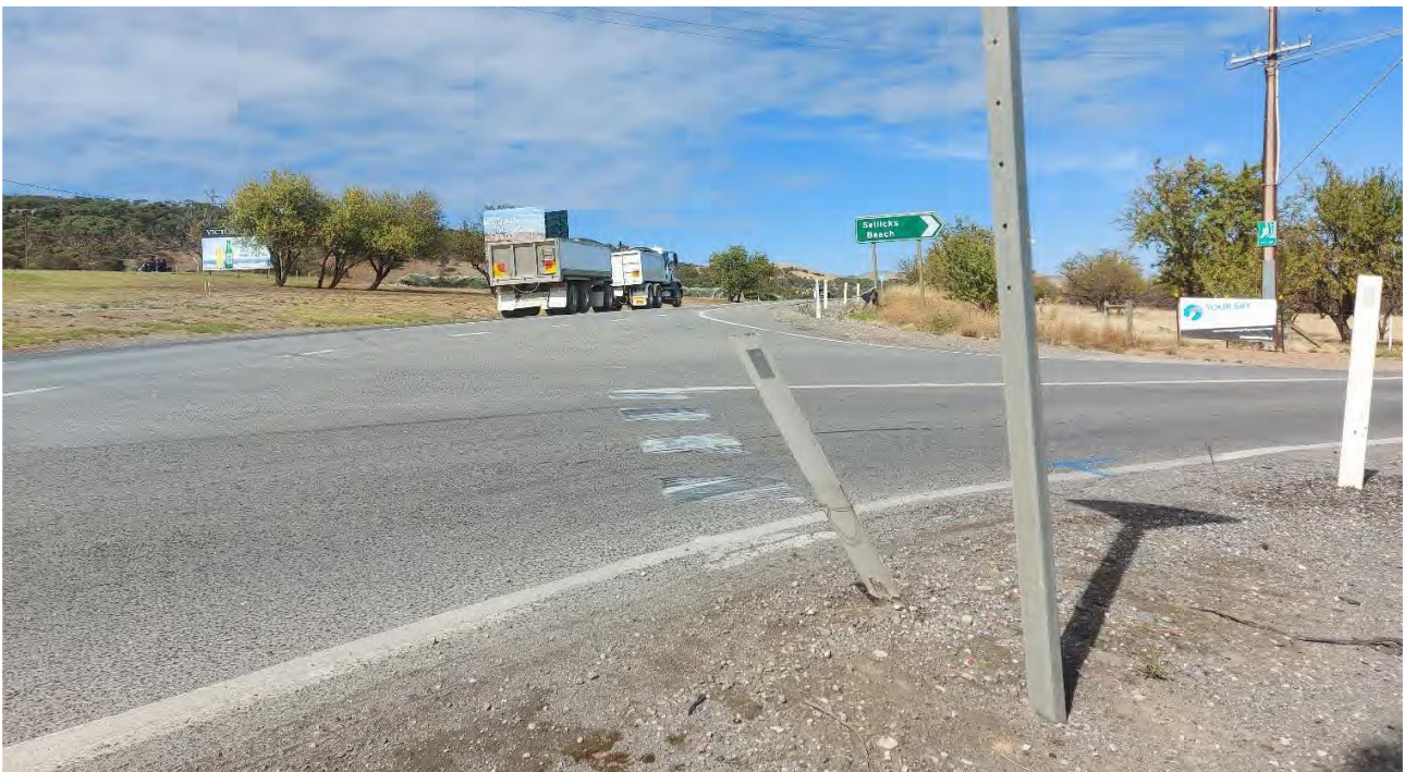
Figure 94: Poor sight distance when turning on to Main South Road from Sellicks Beach Road
