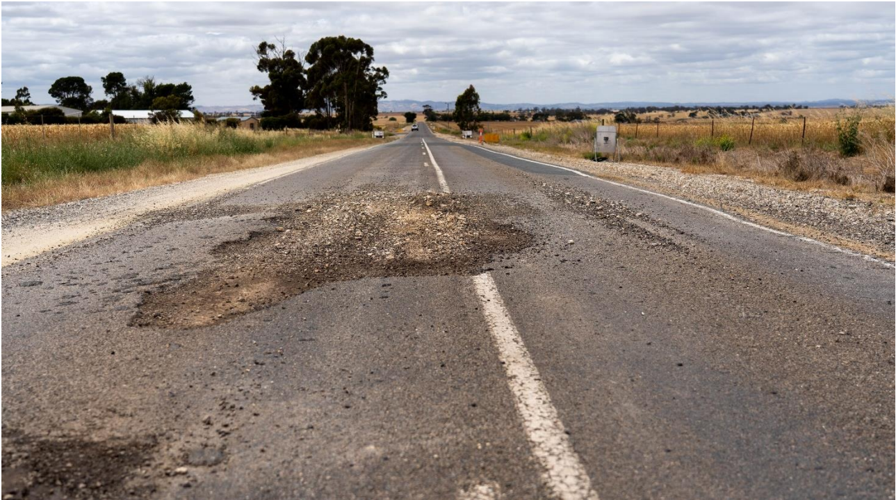
Figure 52: Major pavement failures such as the one pictured above (December 2021) appear regularly on Owen Road
