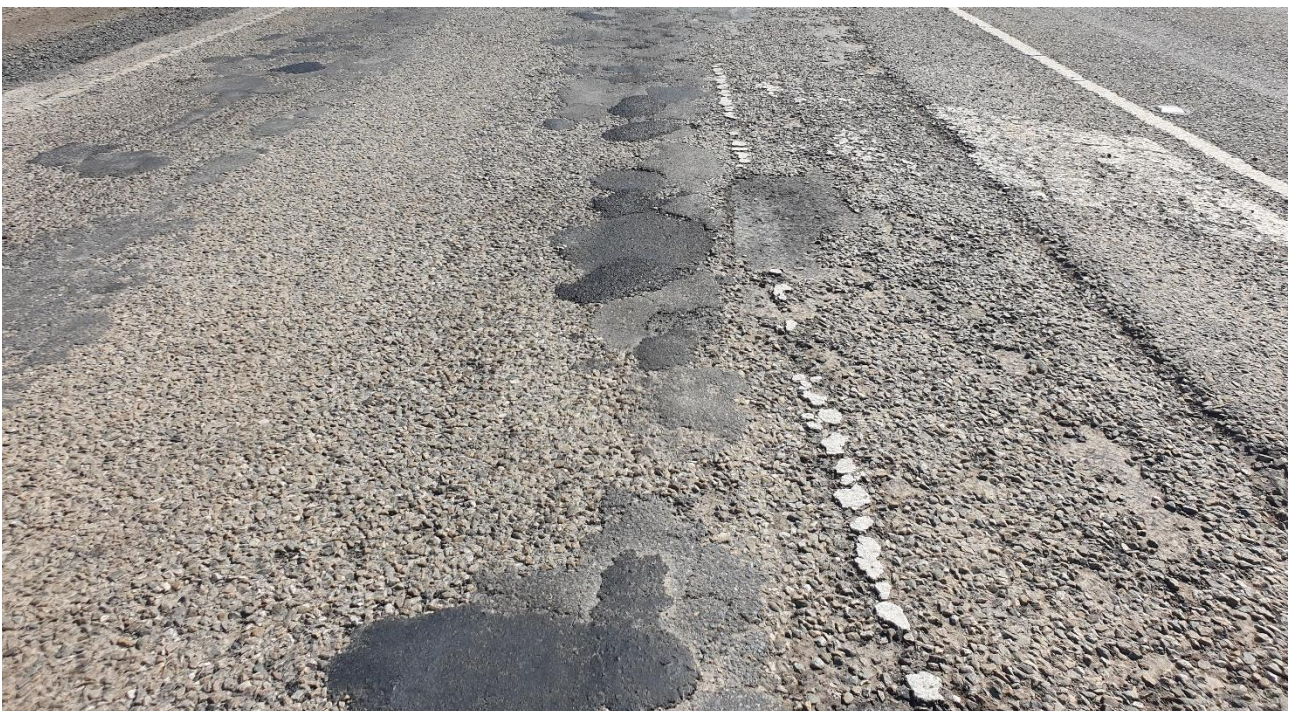
Figure 41: A section of Horrocks Highway between Rhynie and Tarlee assessed by RAA in September 2021
