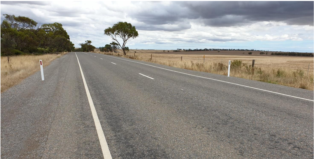
Figure 44: The section between Arthurton and Maitland is significantly safer following an upgrade in 2021
