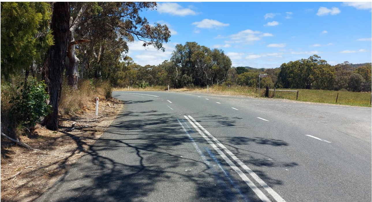
Figure 83: Sight distance is extremely poor when turning right from Strathalbyn Road onto Whites Road
