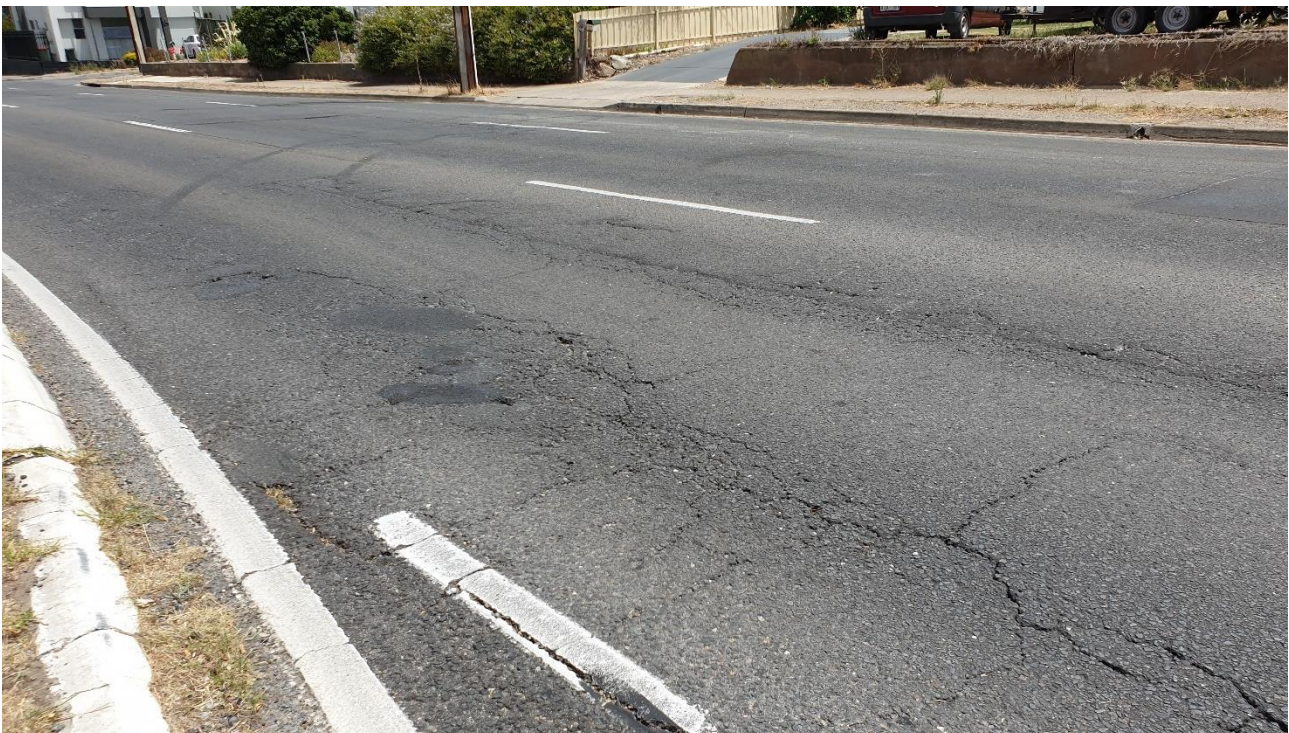
Figure 33: Deteriorated pavement between Golden Grove Road and Hancock Road
