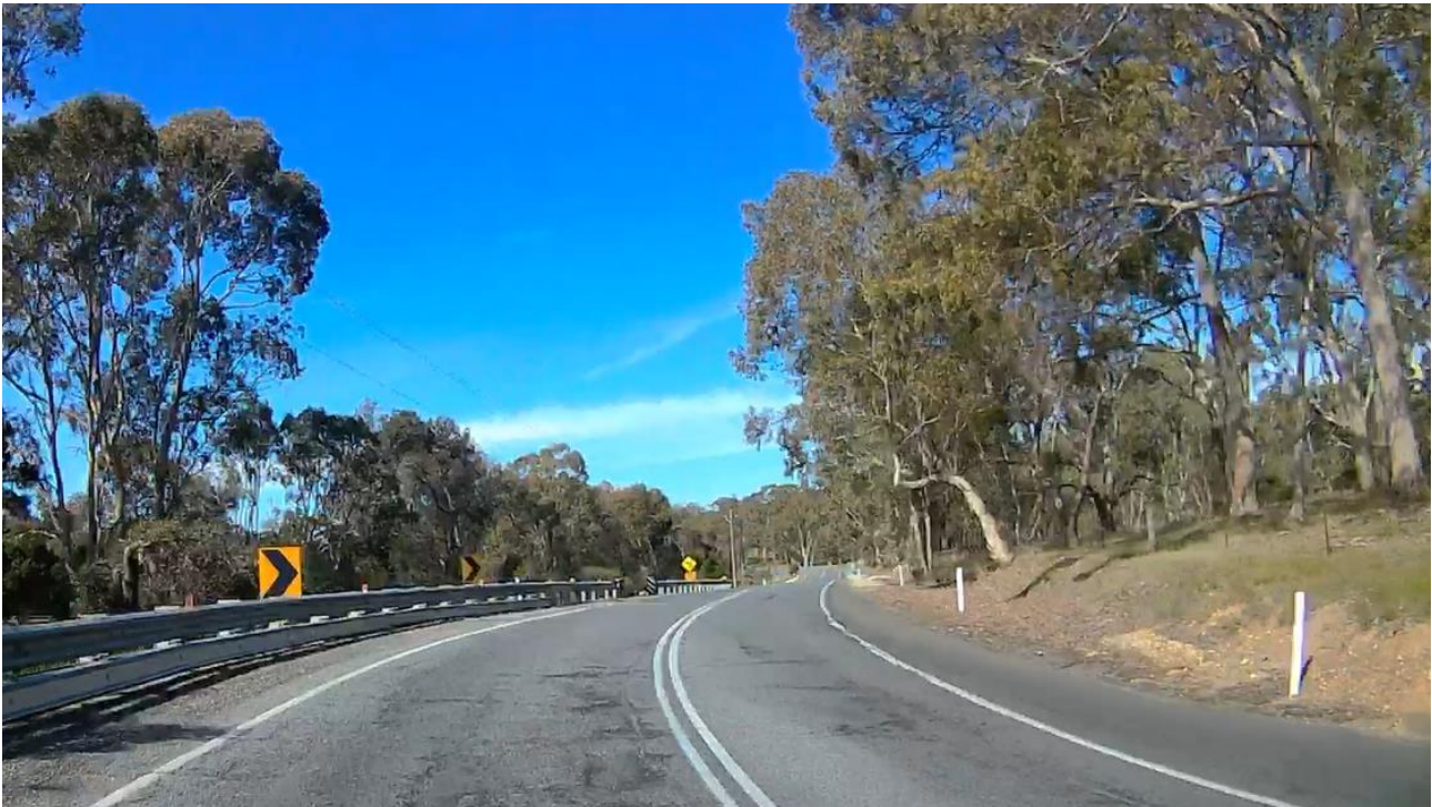
Figure 61: Parts of Torrens Valley Road are in poor condition, which is worse around curves
