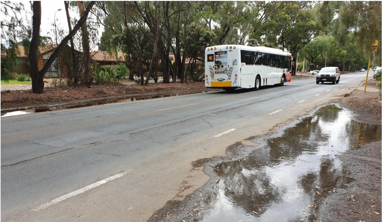
Figure 22: Poor drainage and deteriorated road surface on Kings Road
