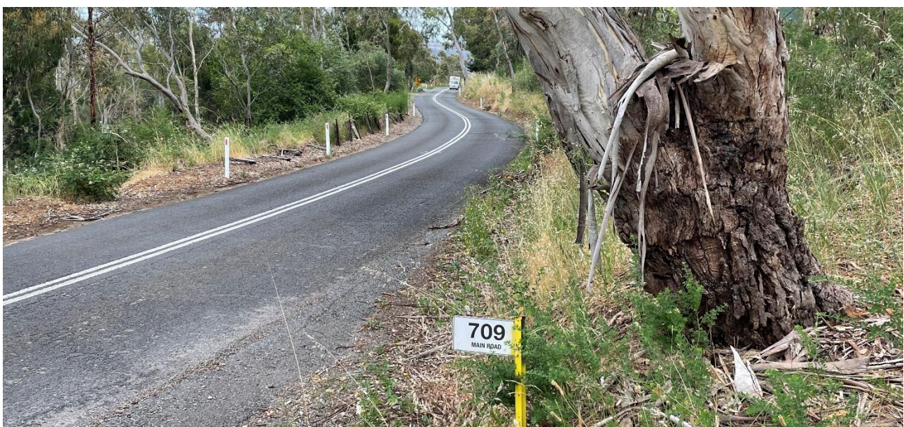
Figure 12: Main Road between Black Road and Oakridge Road is narrow and windy with unforgiving roadsides
